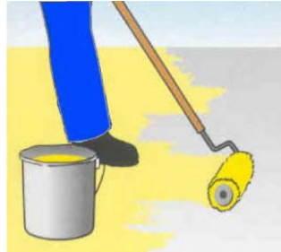
Even application of Primer coat: If moisture content < 4% pbw, prime with SEALER E43 or SEALER E115 . If moisture content > 4% pbw apply (a permanent moisture barrier) system with WETSEAL with medium to long haired roller or brush. E.g. Polyplan roller and brush
